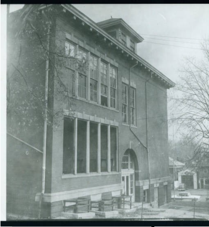
Syracuse Grade School at time of demolition 1956
